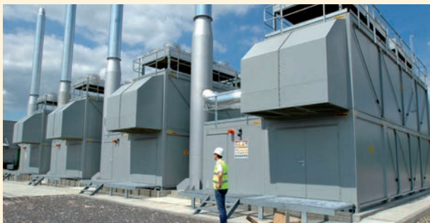
Modulares BHKW – schlüsselfertig Modular combined heat and power station – turnkey
