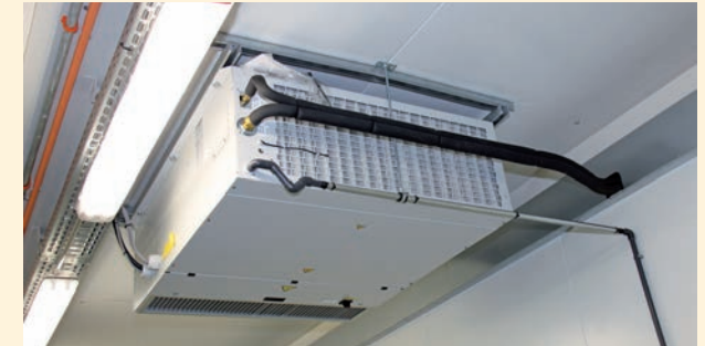
Splitsystem Inneneinheit Split system indoor unit
